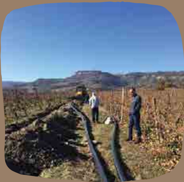
Laying water pipes in Tavush village
